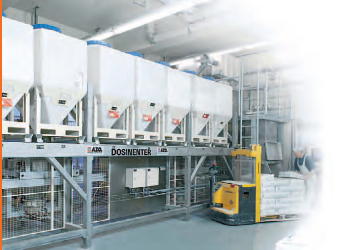
Fully automated weighing with the DOSINENTER® for minor or micro ingredients
