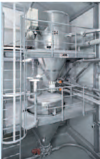
Central weighing system
