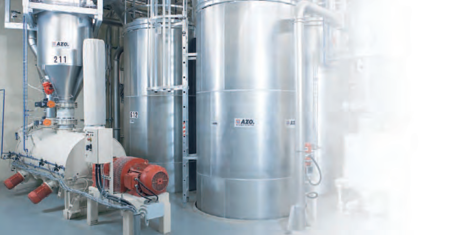
Feeding a horizontal mixer above cooking extruder
