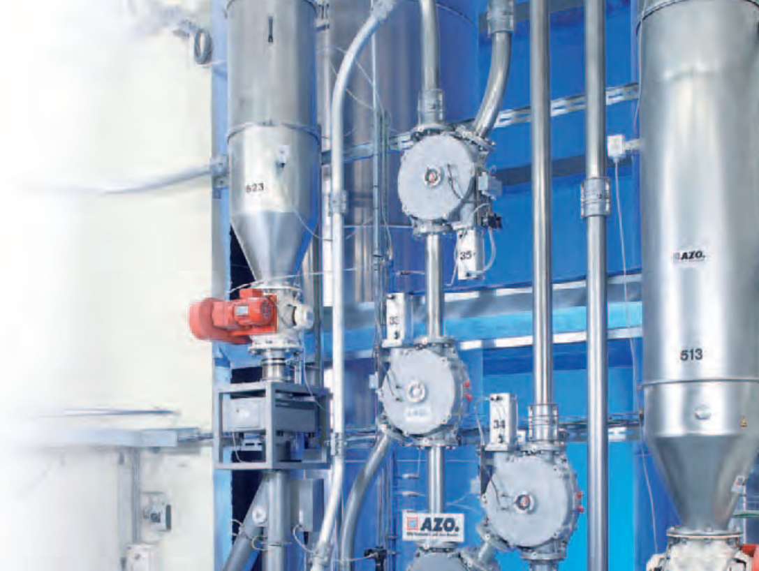
Fully automated metal separation
