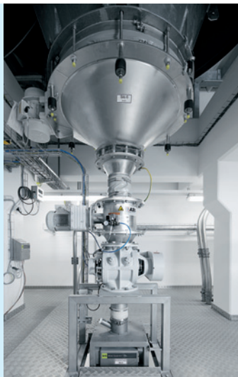
Lump breaker at the outlet from the sugar silo
