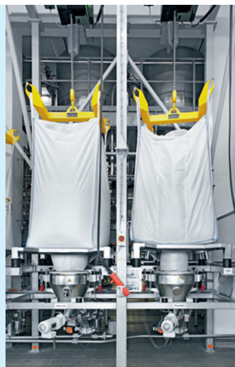
Big bag discharge station for special components
