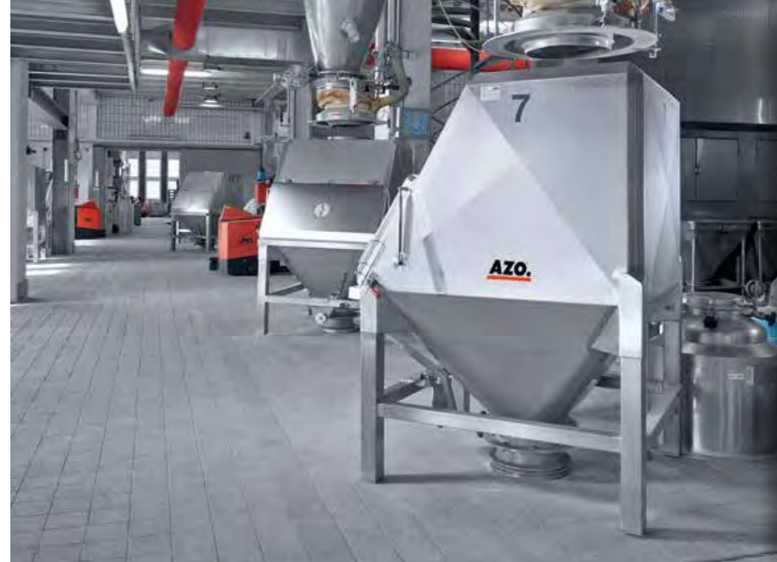
Container docked onto the discharge points above the mixer
