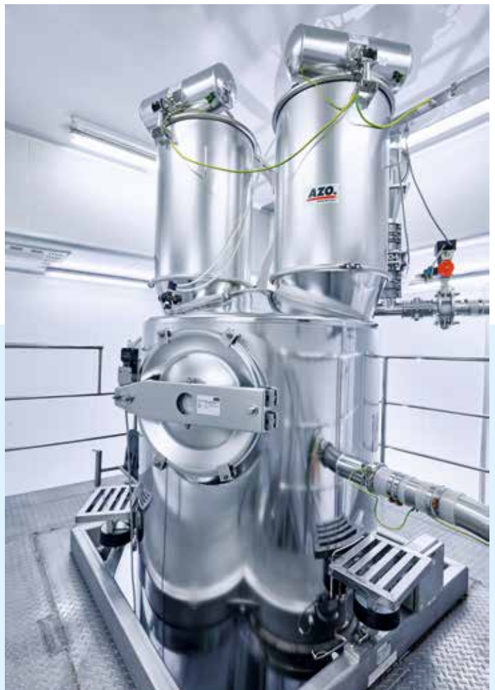
Reliable feeding of the mixer via a vacuum weighing system with conveying scale
