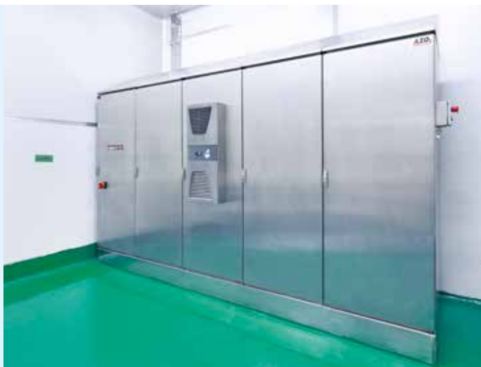
Controls in the MCC room (motor control centre)
