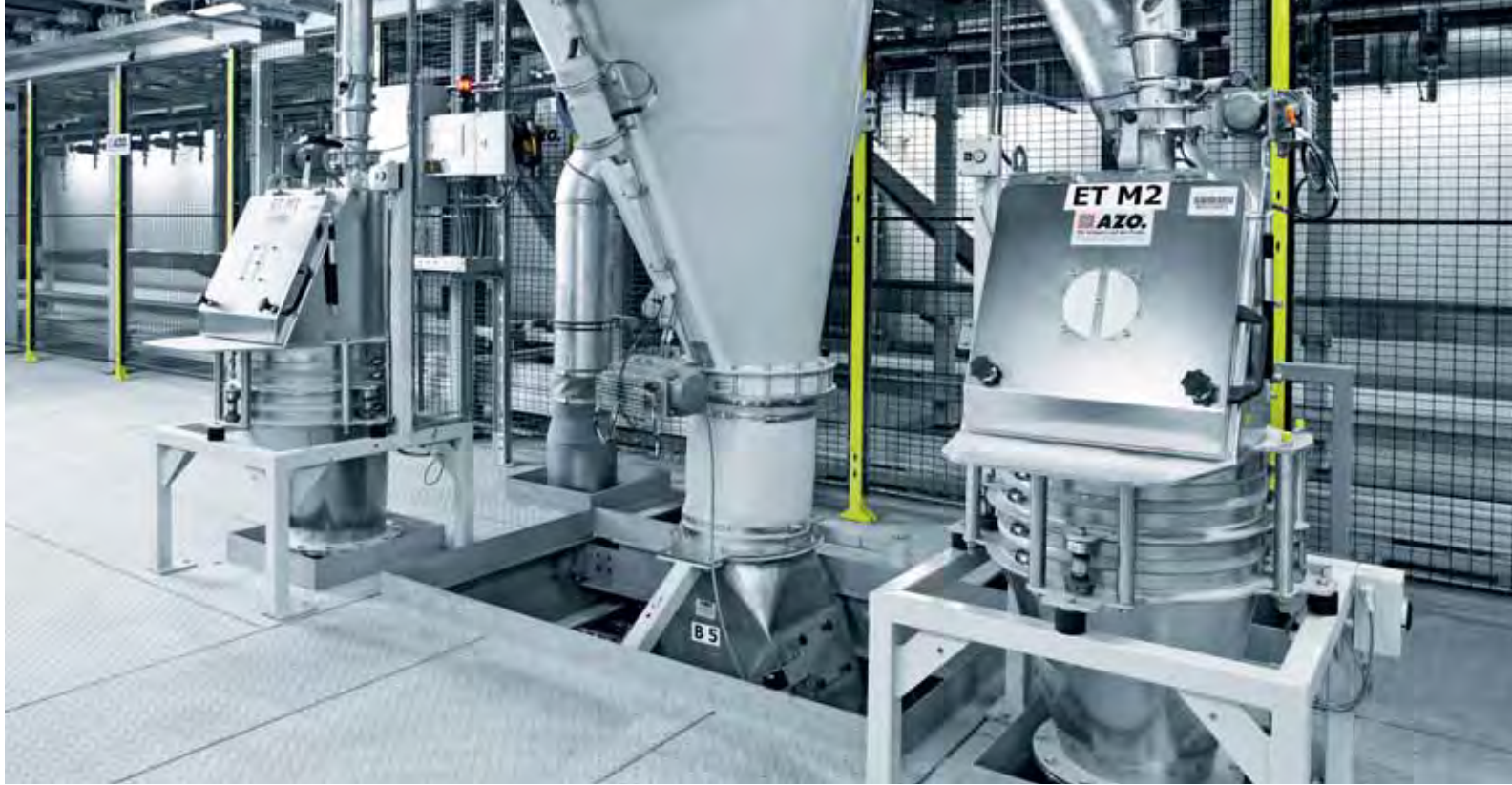
Feeding hopper directly over the mixers for manual additions
