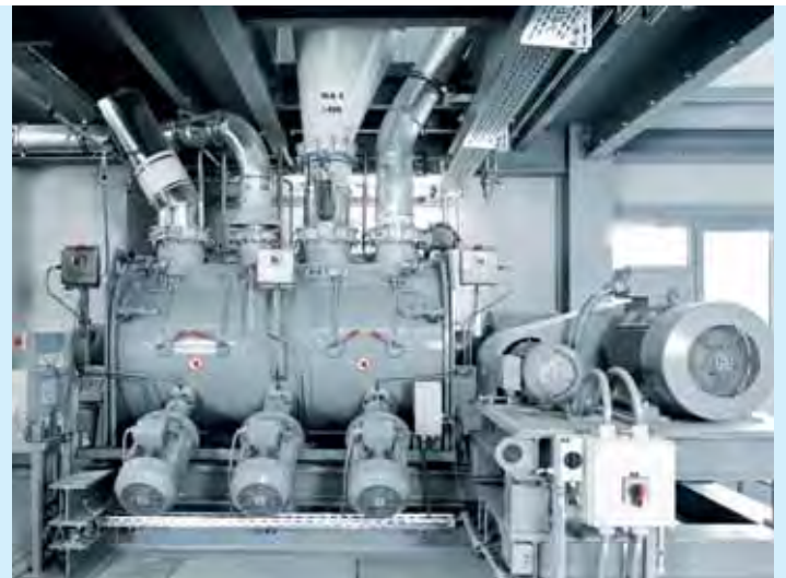
Mixer for making the premixes and special products
