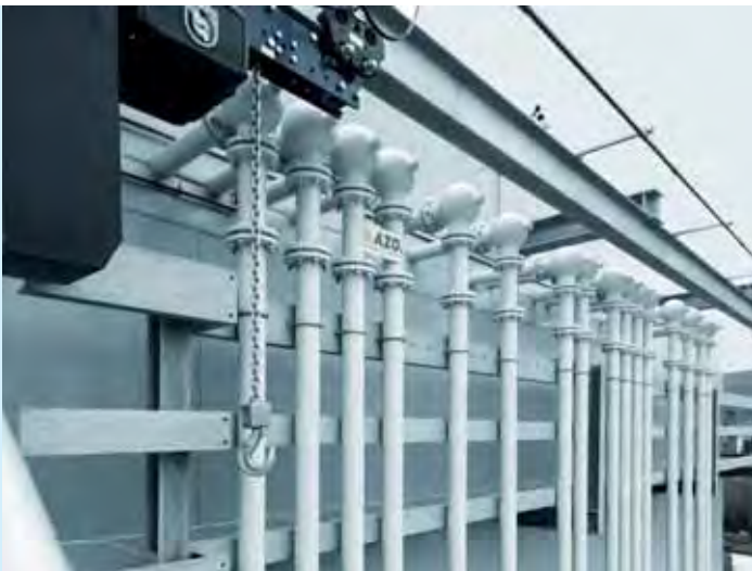
Spherical elbow joints in the filling lines reduce wear and thus extend the replacement intervals
