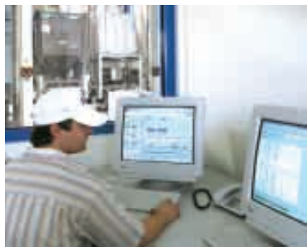
Operation, control, monitoring, documentation
