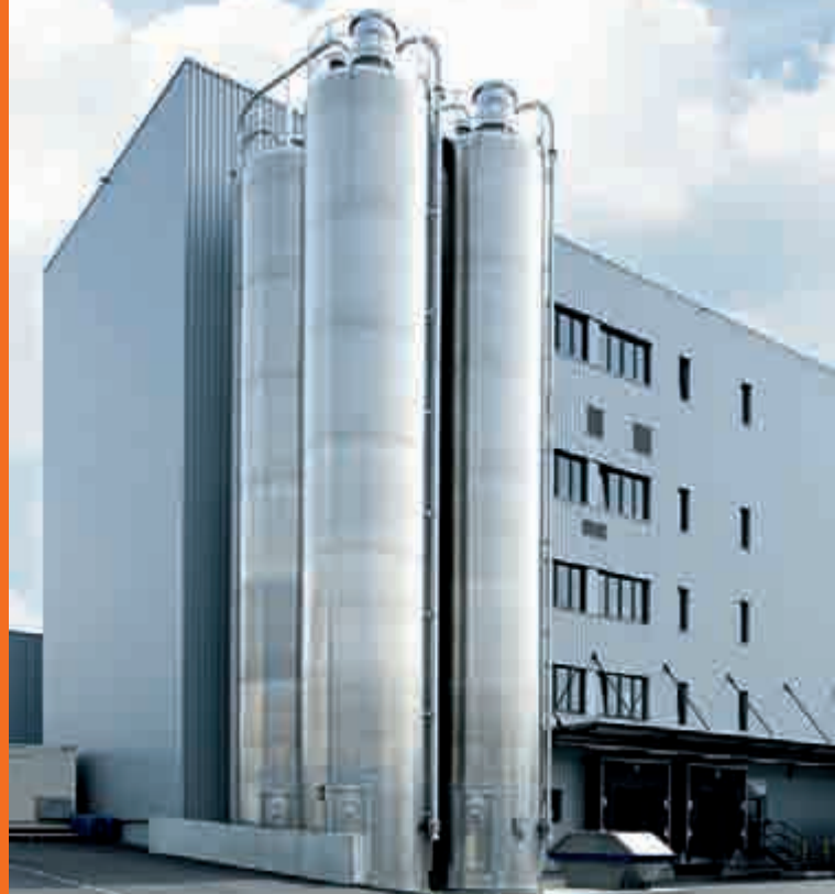
Outdoor silos for large volume storage
