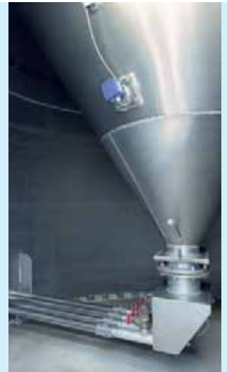
Pick-up cone with four outlets in the silo skirt
