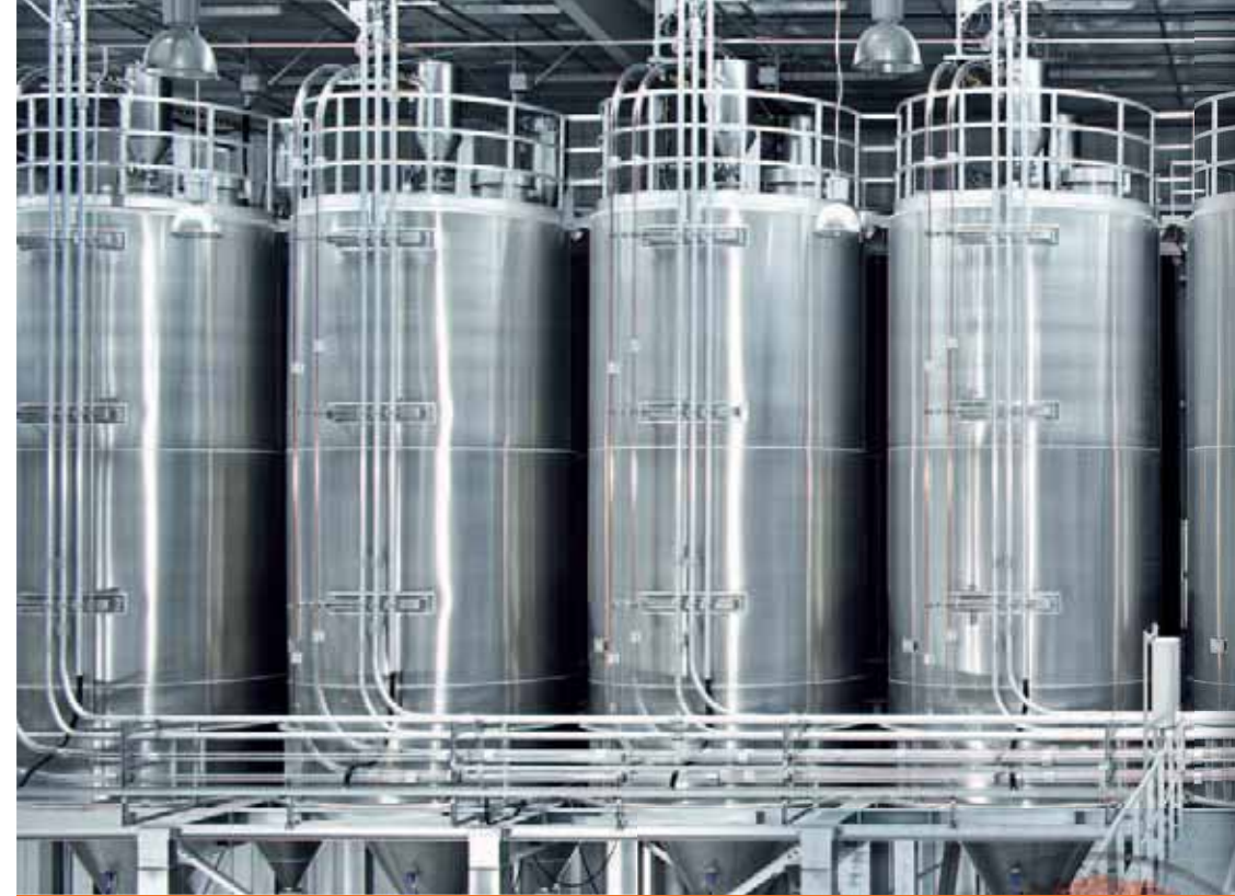
Indoor silos for storing finished goods
