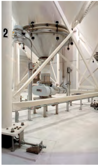
Reliable discharge with vibration bottom
