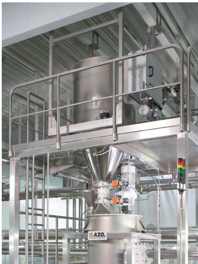
Conveying scales for feeding the kneader lines
