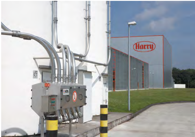
Outdoor silos for storing bulk quantities
