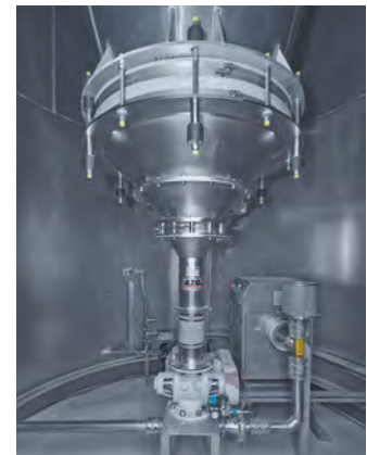
Supply of sugar to the vacuum weighing system with conditioned air
