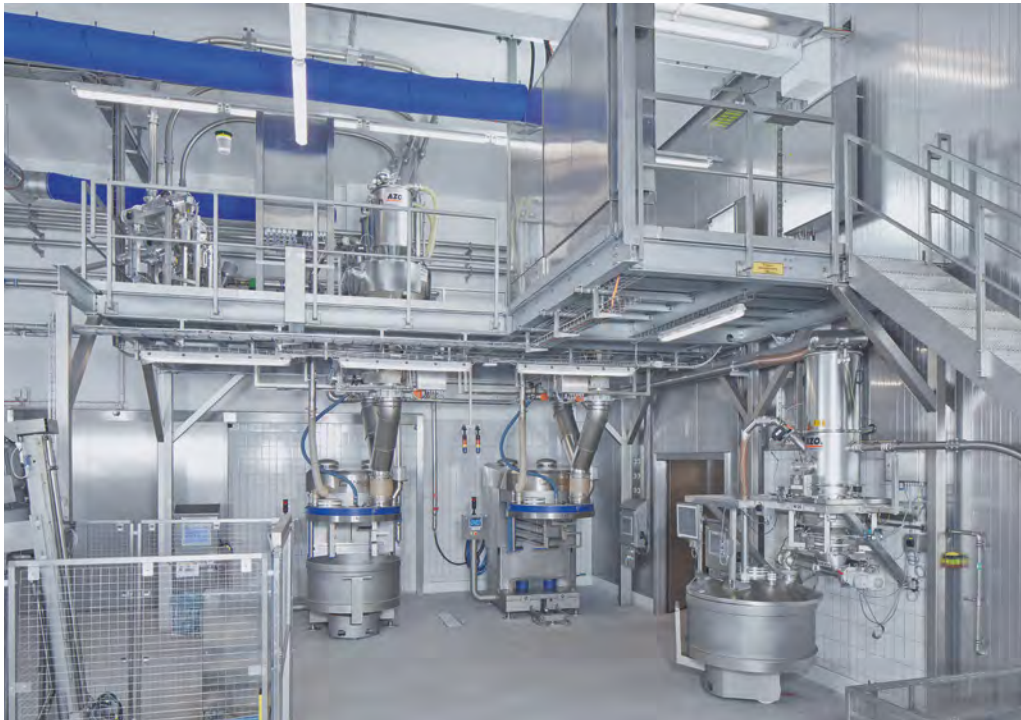
Secure feeding of the kneading lines and little generation of dust as a result of vacuum weighing systems
