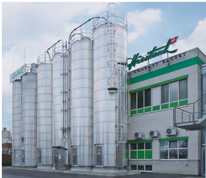
Outdoor silos to store flours and sugar
