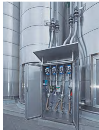
Coupling cabinet at outdoor silos
