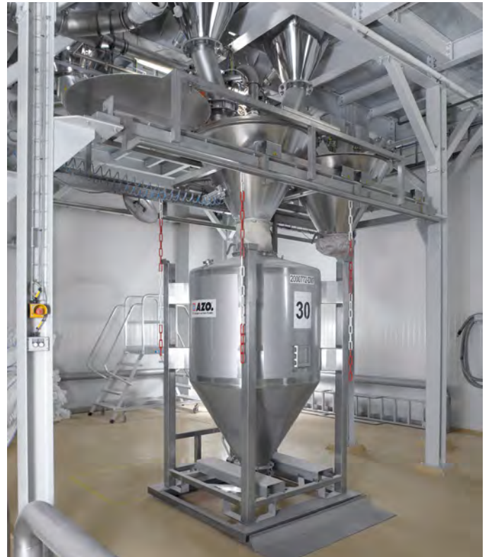
Weighing of light and dark products into BATCHTAINERS® using sliding hoppers
