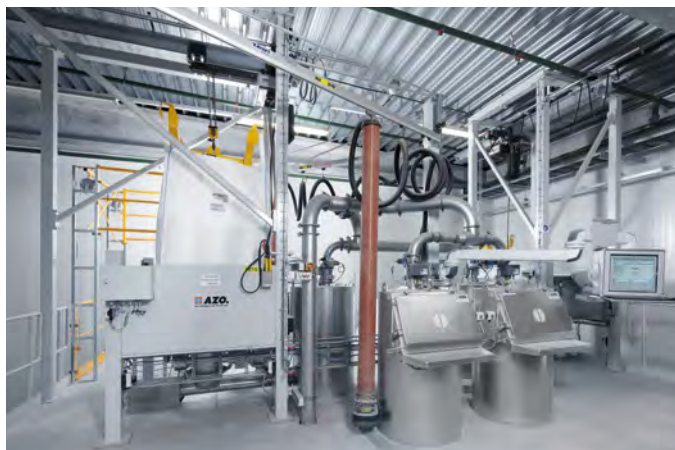
Feeding raw materials via feeding hoppers and big bag discharge stations on the top level
