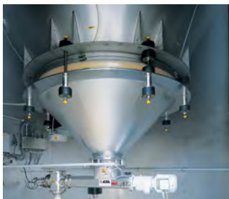
Reliable discharge and dosing
