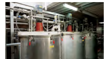
Feeding of dosing vessels
