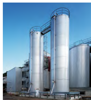
Outdoor silos for kieselguhr
