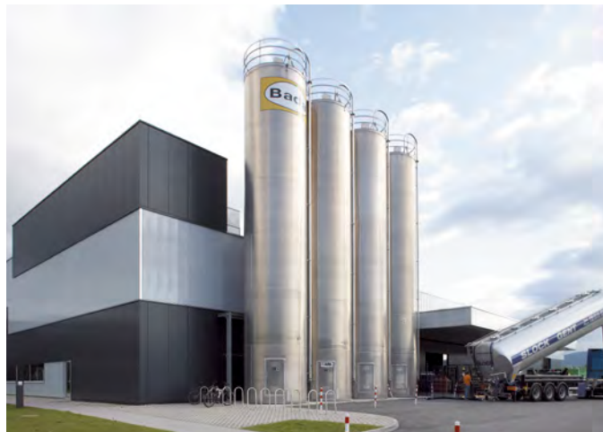
Storing of major ingredients in outdoor silos
