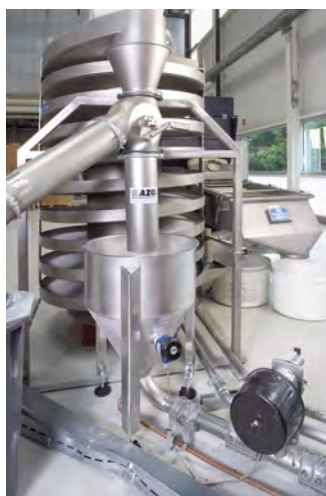
Granulate cooling and feeding of the filling-homogeniser silos
