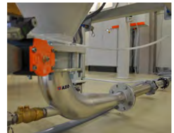
Supply of the product into the transport line
