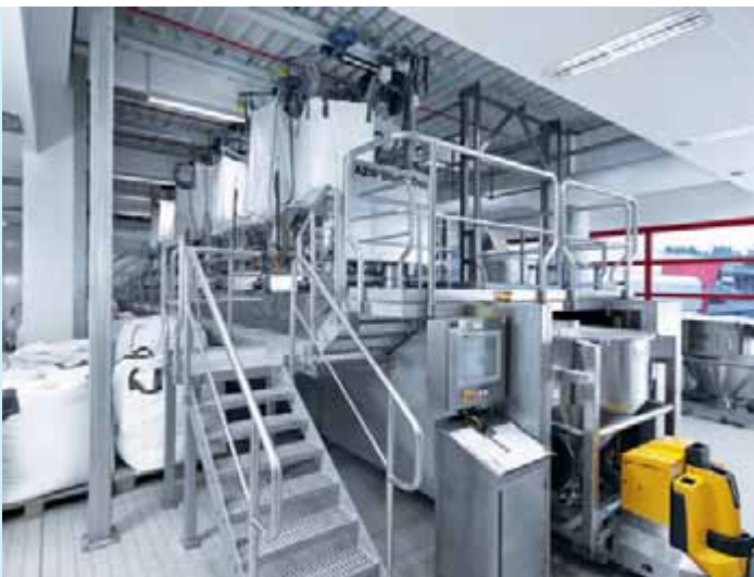
Transfer of an AZO MIXTAINER® in the dosing line
